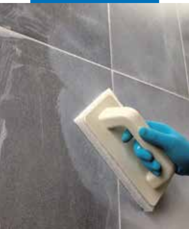
Cleaning the joints with a Scotch-Brite® pad
