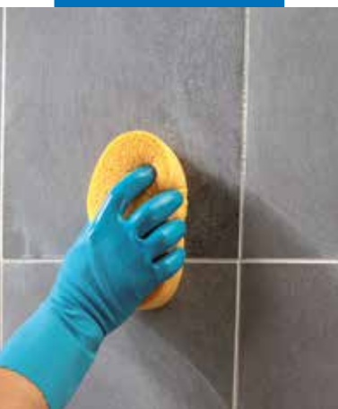
Finishing the surface with a hard cellulose sponge
