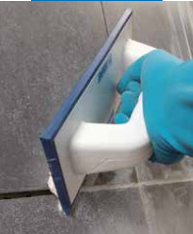
Application of Flexcolor with a rubber trowel
