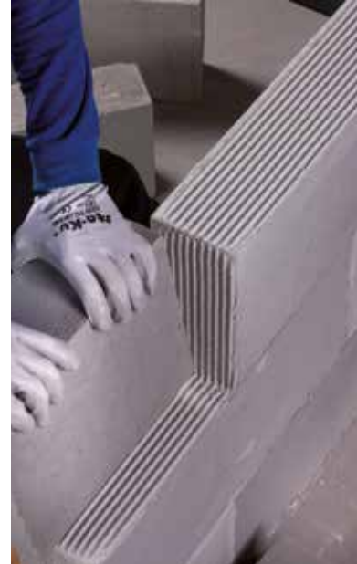
Laying blocks on Porocol FF still fresh
